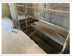
Red tape does not serve as fall protection. A guard rail should be posted here.
