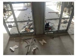
Debris and materials are blocking the access way. The materials should be cleared from access ways and trash disposed of.
