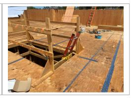
Example of offset wall used for a ladder opening.
