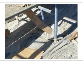
Platform incomplete. Ensure planks are replaced.
