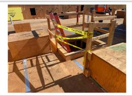
Ciarra employee reminded of proper ladder use. A-frame ladders should not be leaned against the wall. They must be opened for proper use.
