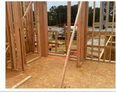
At the garages, an employee was working off a folded step ladder. Ladders must be opened and used as intended.
