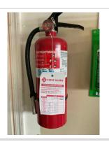
Roofers were using flammable gases and liquids, but did not have a fire extinguisher within 25 feet of those materials.
