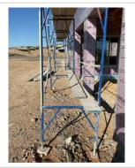
There must be no gaps greater than an inch in between planks.
