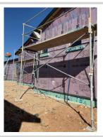
Must not use severely damaged planks or damaged pads for mud sills for the baseplates on the scaffolding.
