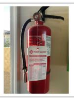
Framers were using flammable gases and liquids, but did not have a fire extinguisher within 25 feet of those materials.
