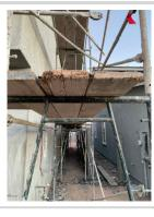
All sections of scaffolding should be fully planked and there should be no gaps greater than an inch in between planks.
