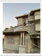
Guardrails should never be removed from the scaffolding, the guardrails are apart of the scaffolding structure.
