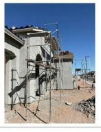
Single planks used on scaffolding is prohibited. Must have a minimum of three planks .
