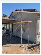
All sections of scaffolding must be fully planked and there should never be any gaps greater than an inch in between planks.
