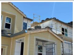
Lot 75: Scaffold railing on upper section has been removed and left hanging. All scaffold railing must be maintained at all times. Do not modify scaffold without supervision of scaffold competent person and erector.
