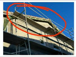
The scaffold on lit # 1039 the planks are not overlapping and there is a gap
