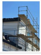
Scaffold erected inside home needs guard rails at second level and has to single planks used for access at second floor level. Planks need to be removed and not used, as it is not adequate to protect from falls.
