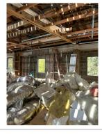
Access ladder was extended 3 ft but should be secured if in use
