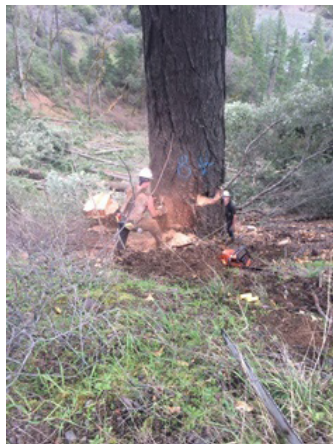
Trained loggers had to fell huge trees on a 10-acre parcel to clear the way for the viaducts.
